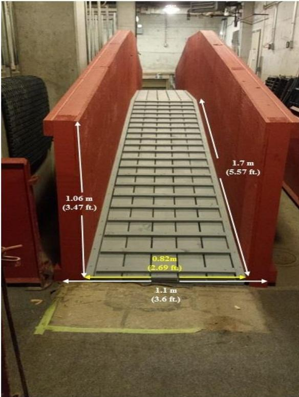
Figure 3: Walkway section of ramp
