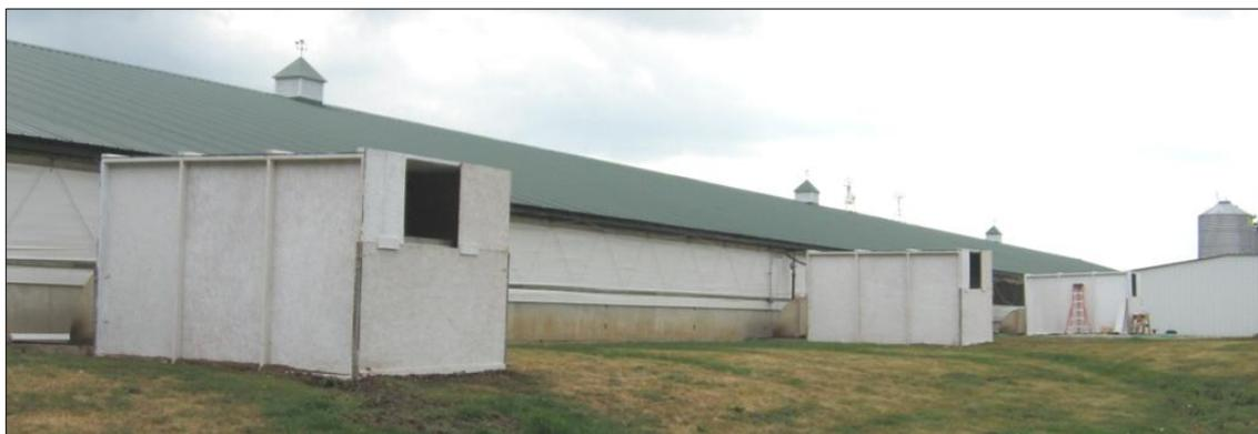
Figure 2. Enclosures installed at pit fans 1, 2 and 3 to collect and redirect the biofilter-treated (fan 1 = biofilter 1, fan 3 = biofilter 2) and untreated (fan 2 = enclosure 2) exhaust streams.
